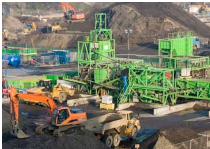
First aid: A 'soil hospital' was set up to clean the most contaminated soil
